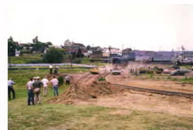
After Engine 225 was in place, crews repeated the process with Tender 236.
