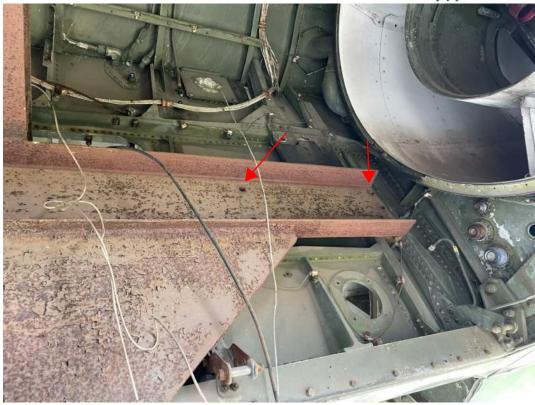
Photo 5: Interior of the connection – looking north on east side of the column – Note the missing bolts at the ends of the steel channels which are supposed to transfer loads from the aircraft frame to the support.
