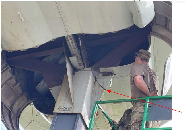
Photo 3: Exterior- View looking east at the failed south gusset on June 12, 2023.
