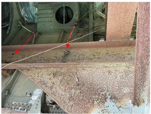
Photo 6: Interior of the connection – looking north at west side of column– note only one bolt remains connecting the weldment to the aircraft.
