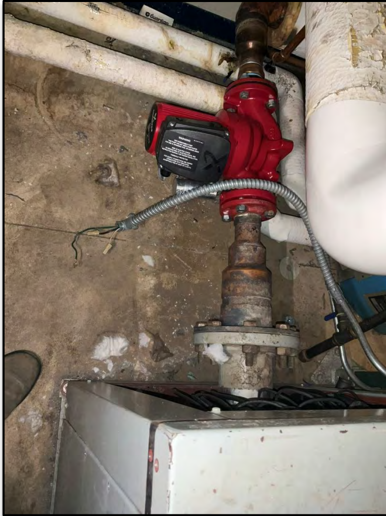
Figure 1: New Pump Installed
