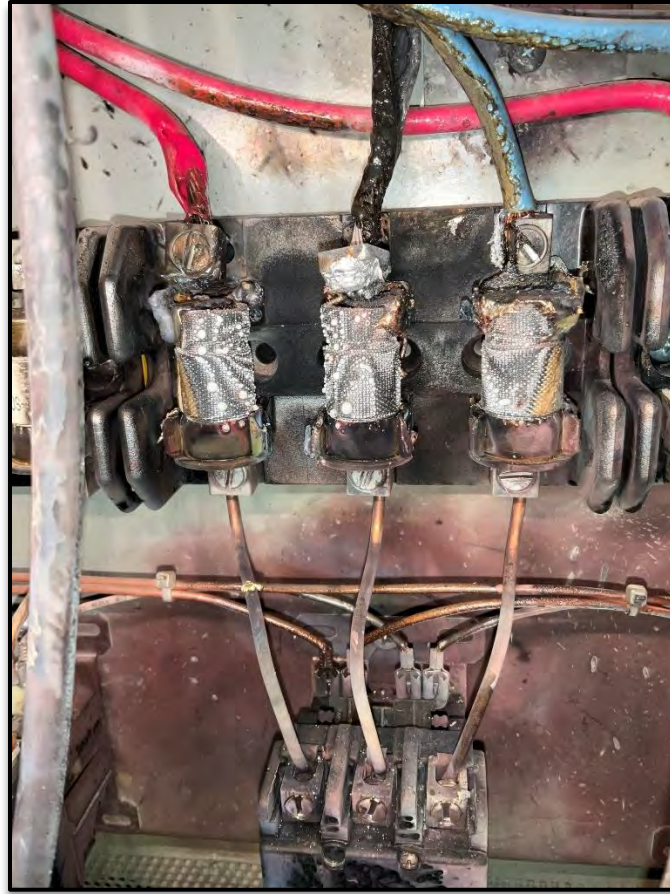
Figure 3: Arcing event between fuses
