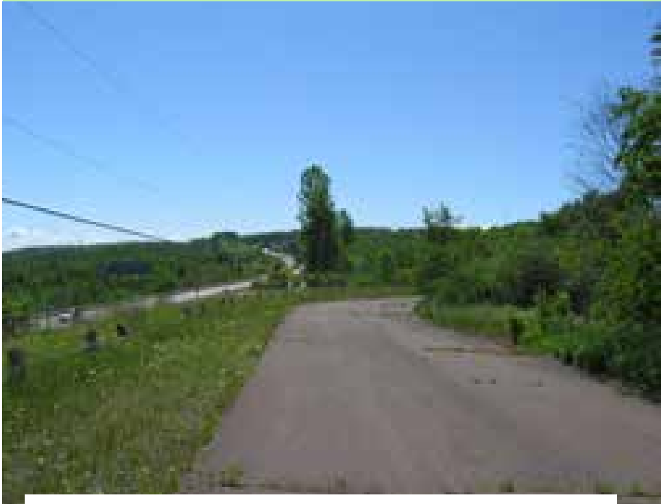
Old Hwy 61 – good condition of old roadway
